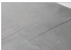
Back cracks
